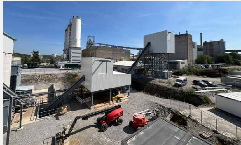
Alternative fuel plant after completion
