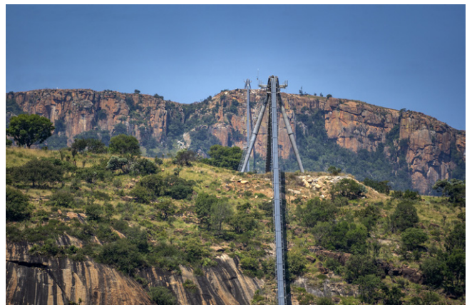
Doppelmayr_BooySendalSouth_01.jpg - The RopeCon® easily crosses this topographically challenging terrain.
