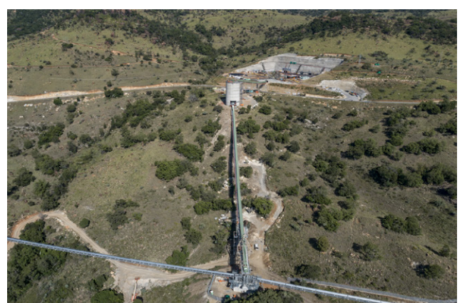
Doppelmayr_BooySendalNorth_01.jpg - The option of an alternative loading point was provided at tower 2
