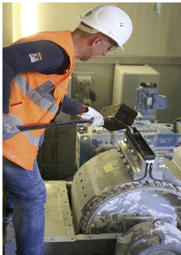
Picture 3: After casting, the junction is cured very quickly.
