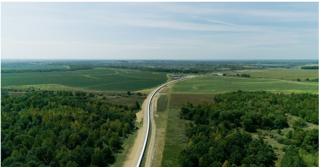
Picture 2: A 6.5 kilometre long overland conveyor for coal: The concept of only one conveyor prevailed against four straight conveyors with transfer towers.
