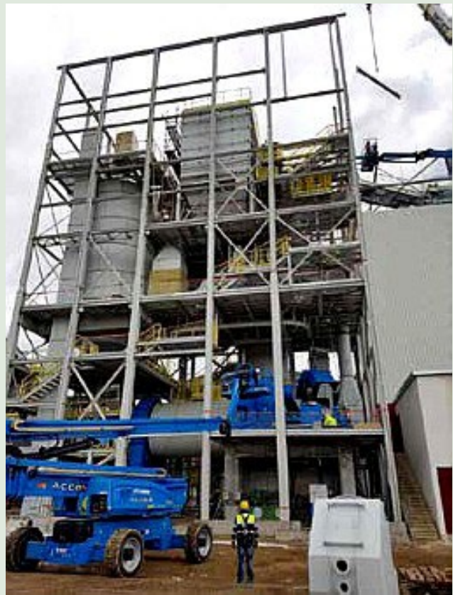
Steel construction of the grinding module.
