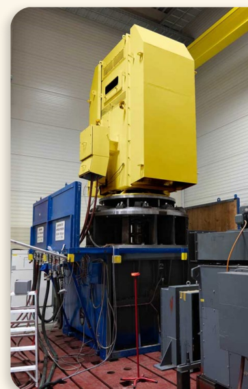
Menzel Elektromotoren now also performs load tests on large industrial motors in a vertical installation position
