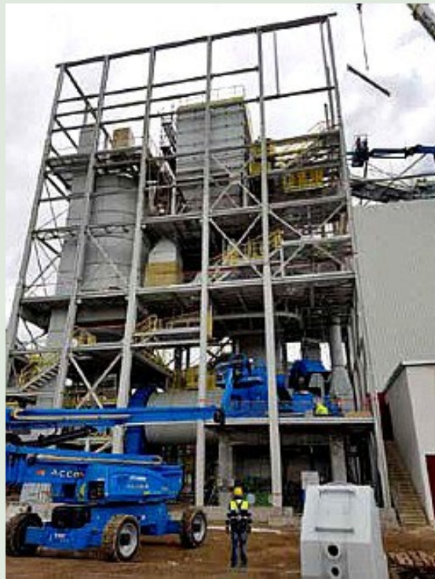
Steel construction of the grinding module.
