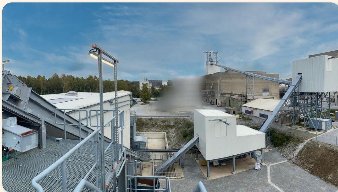
Alternative Fuel Plant in operation since Q1 2025
