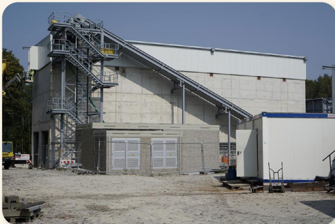
2. AF (alternative fuel) storing with automatic reclaimer
