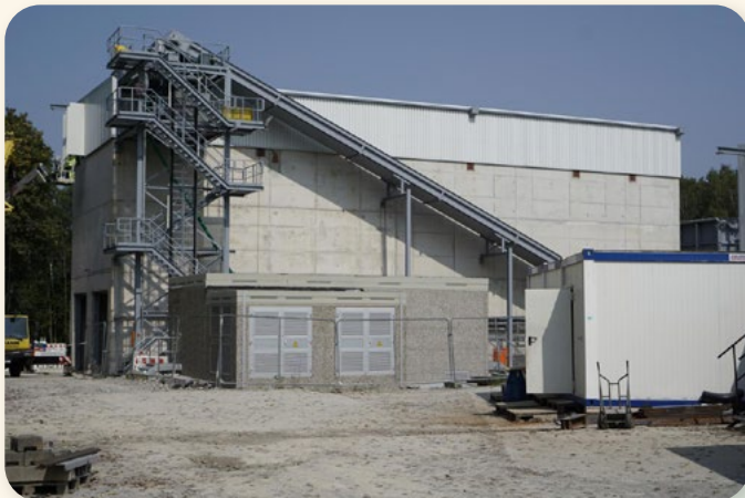
2. AF (alternative fuel) storing with automatic reclaimer
