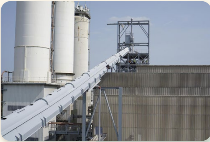
5. Air-supported belt conveyor
