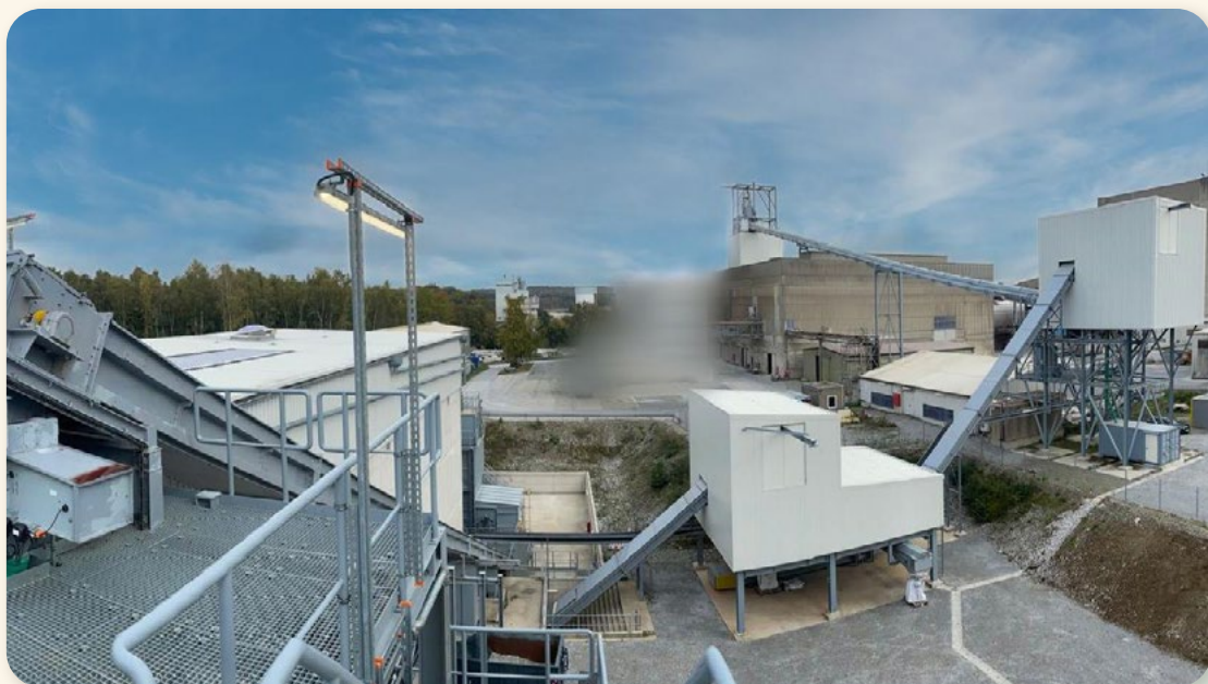
Alternative Fuel Plant in operation since Q1 2025
