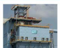
ESP TO BAG FILTER CONVERSION
