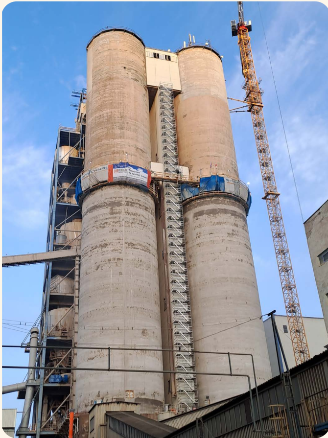
Silos during slipform procedure
